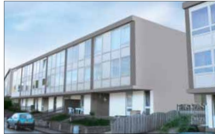
Vrieheide low income residences after renovation.
