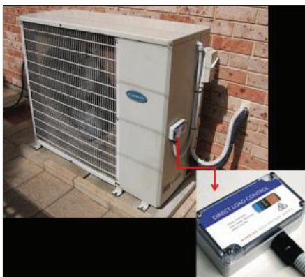
► Figure 3. Saab Systems “Peak Breaker” Direct Load Control Device Used in the ETSA Utilities Air Conditioner DLC Phase II Project
