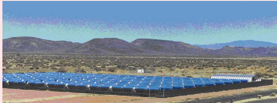
Figure 41: A monthly bill is issued to a prison for actual energy delivered by a large solar water heating system in Phoenix.
