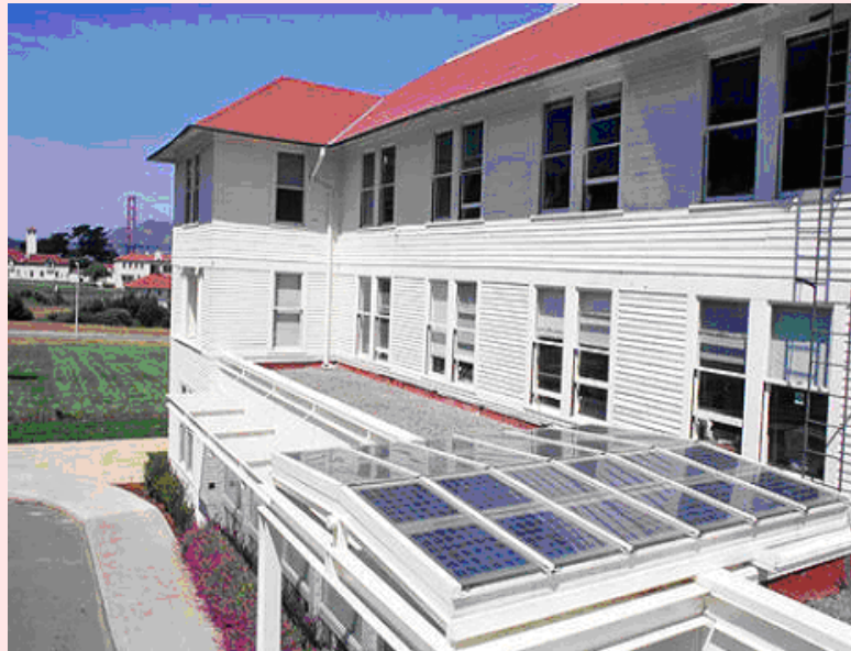
Figure 45: Building-integrated PV system in the Presidio, San Francisco.
